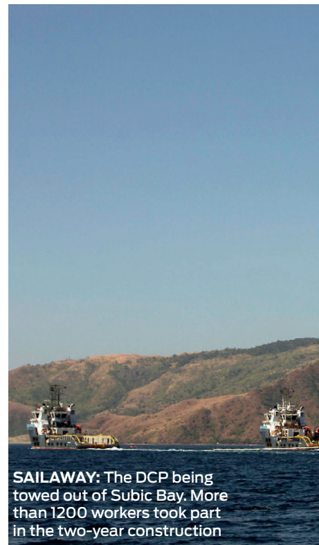
LOCAL CONTENT: The DCP, under construction at Keppel's Subic Shipyard, has 80-metre legs that are jacked down for self-installation.
