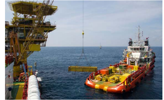
Transfer Well Workover equipment onto platform, using platform supply vessel (PSV)
