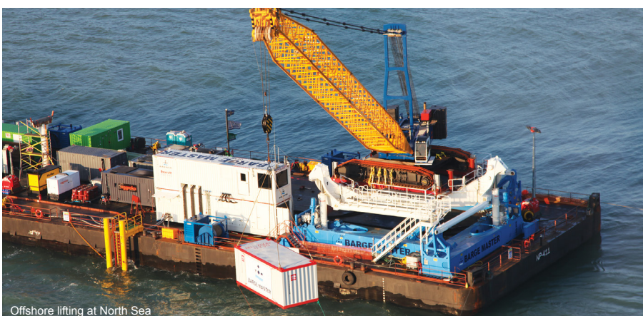
Offshore lifting at North Sea
