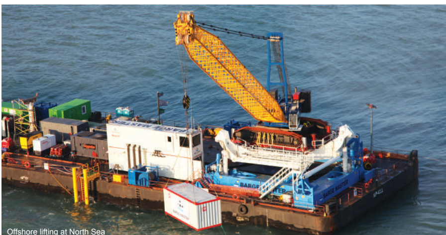
Offshore lifting at North Sea
